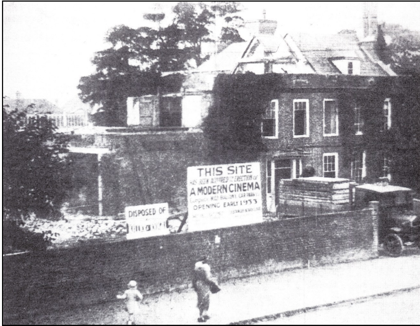
Demolition of part of Ravenswood 1932 for a cinema
